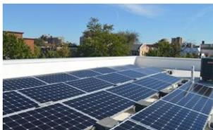
In partnership with Enterprise and the Sustainable Energy Utility, the National Housing Trust installed solar panels on 11 multifamily affordable buildings in Washington, DC. The systems will reduce operating expenses by over \$27,500 per year on and offset over 100,000 kWh from the electric utility supply grid. The money saved from **energy efficiency helps preserve affordable rents and maintain resident services**, like tutoring programs and financial education.
